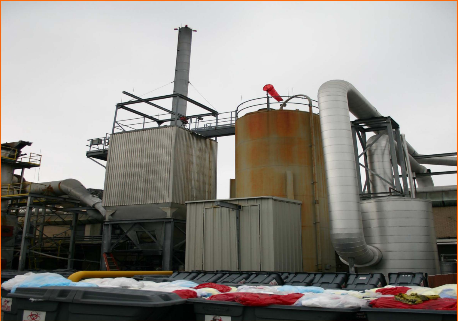
St. Joseph's Hospital Incinerator Tampa, Florida
